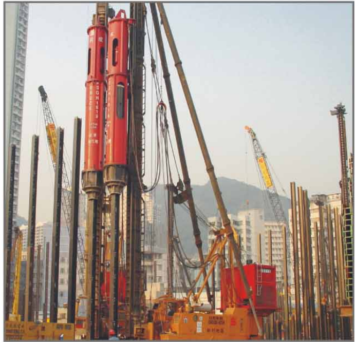
BRUCE SGH-1618 & 1619 in Hong Kong driving H-beam piles (305mmx 305mm, 223kg/m, 48m long)
