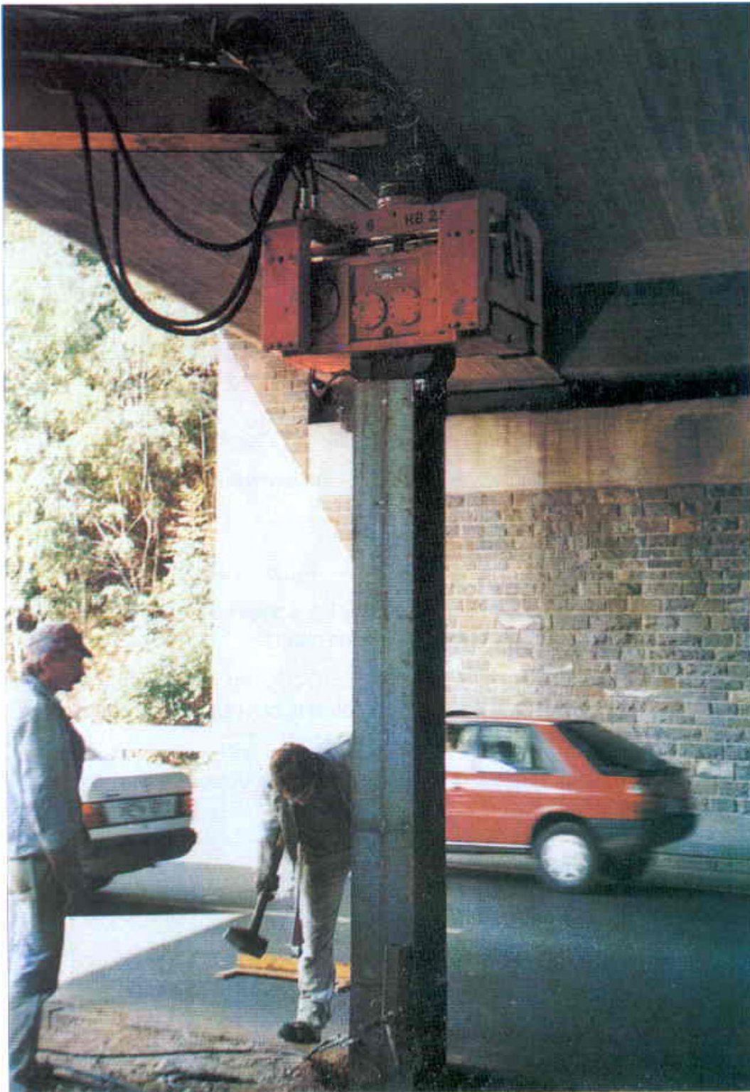
Figure 10.2-4: If the soil conditions allow the use of vibrators fixed directly to the boom of an excavator this may be a reasonable solution, as shown in the picture.
